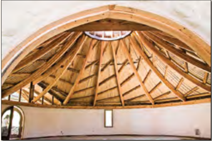
Note that the central steel tension ring not only holds the rafters securely in place (they're bolted), but creates a large circular skylight, a light-infused mandala.
