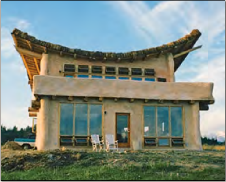
Timber frame of fir and hemlock, wrapped with plastered straw bales
