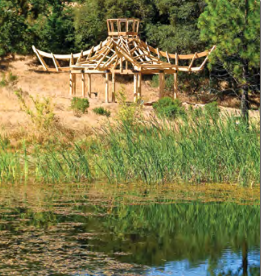
Temple under construction in Northern California hills, a small version of the temple on pp. 64-71. Twelve-sided, 33 feet in diameter. Entrance will be to the east, fireplace to west; walls will be straw bales and cob.
