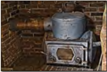
Wood-fired boiler for radiant heating
