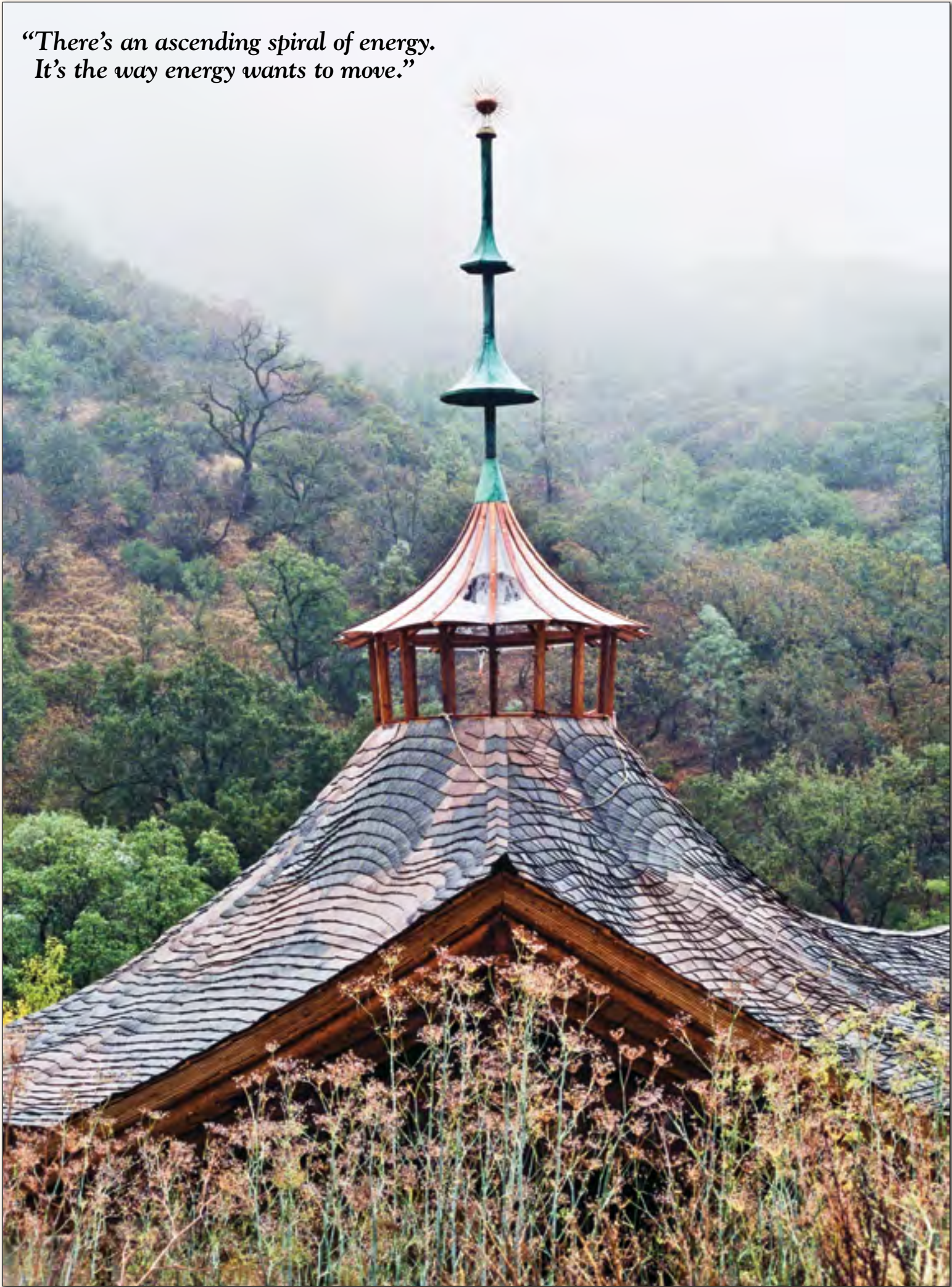
At the apex of the temple is a 16-sided cupola, with outward-slanting walls. There are motors that open every other window
