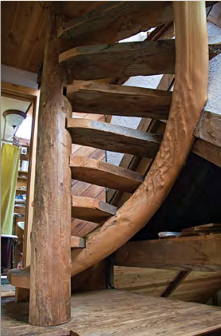
Improvised spiral staircase with curved log
