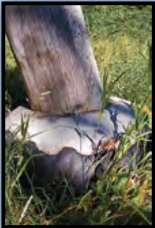
Foundation anchor: tractor tire filled with concrete
