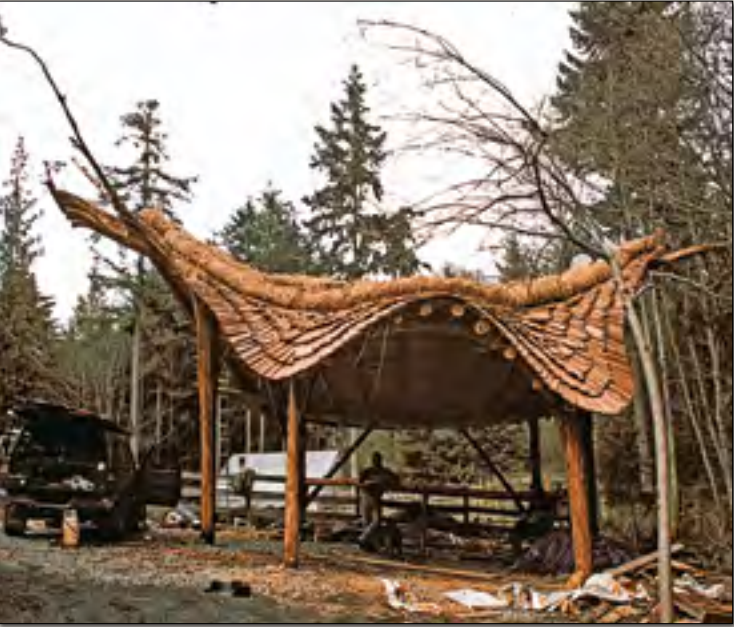
Pavilion, 20' long, 16' high, is on Whidbey Island, Washington. All framing was fir from property.
