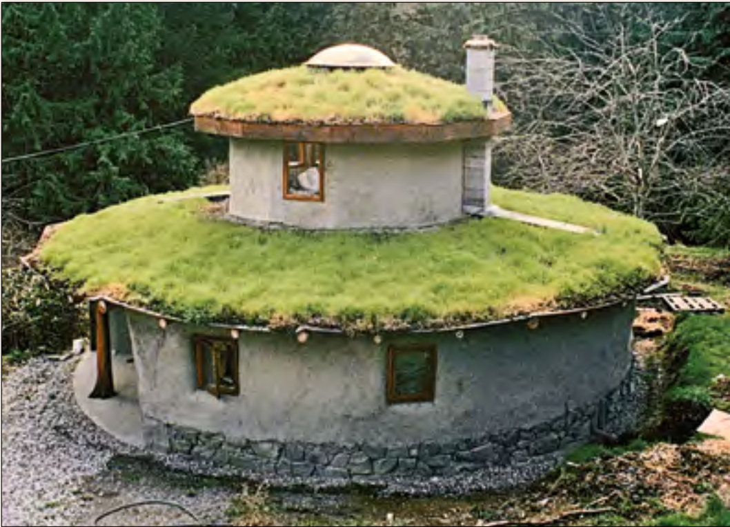
Kai’s straw bale house uses pond liners under the sod roofs.
