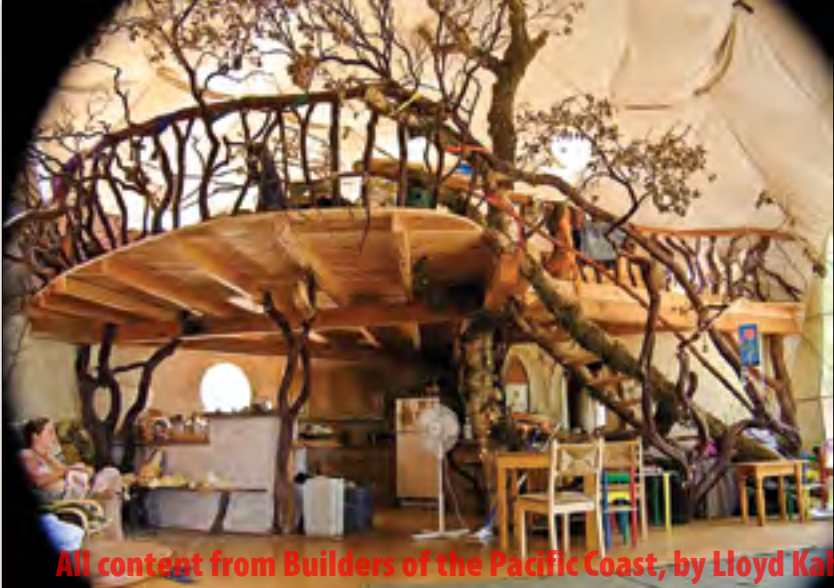
Loft in geodesic dome. Live oak supports loft, with manzanita railing harvested from property
