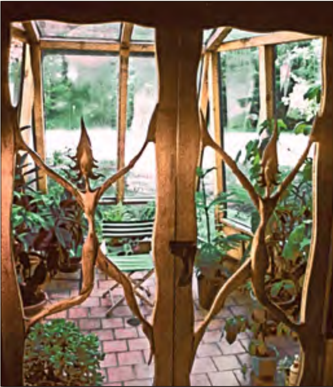
Door for John Knudson's house is wood glued to sheets of glass.
